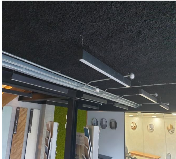
Office in Dublin, Ireland
