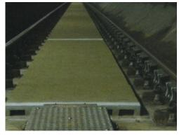
Smaller panels installed at the sides to hide fixings. Plugs of the same material hide the screw holes.
