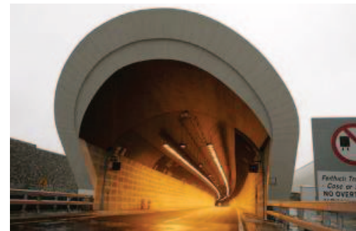
Quietstone Light clearly visable on the entrance to the tunnel
